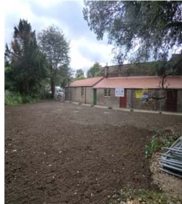
Top soil grading at Bothies
