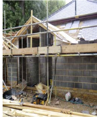
West Stable block extension
