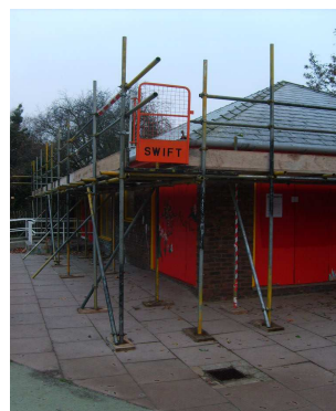
Rainbow Hut Roof Removal
